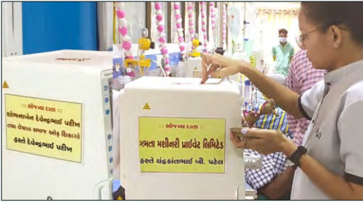
Two more Dialysis machines installed at Sanjivani
